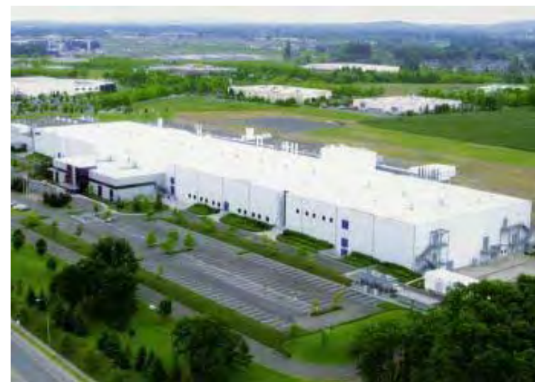
SolarWorld (landscape buffer and parking) (Source: http://solarhope.wordpress.com/2007/03/ )
